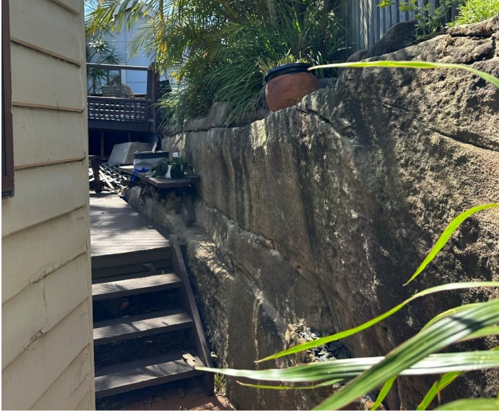
Figure 9. View to rear decks and adjacent rock outcrops to be removed.
