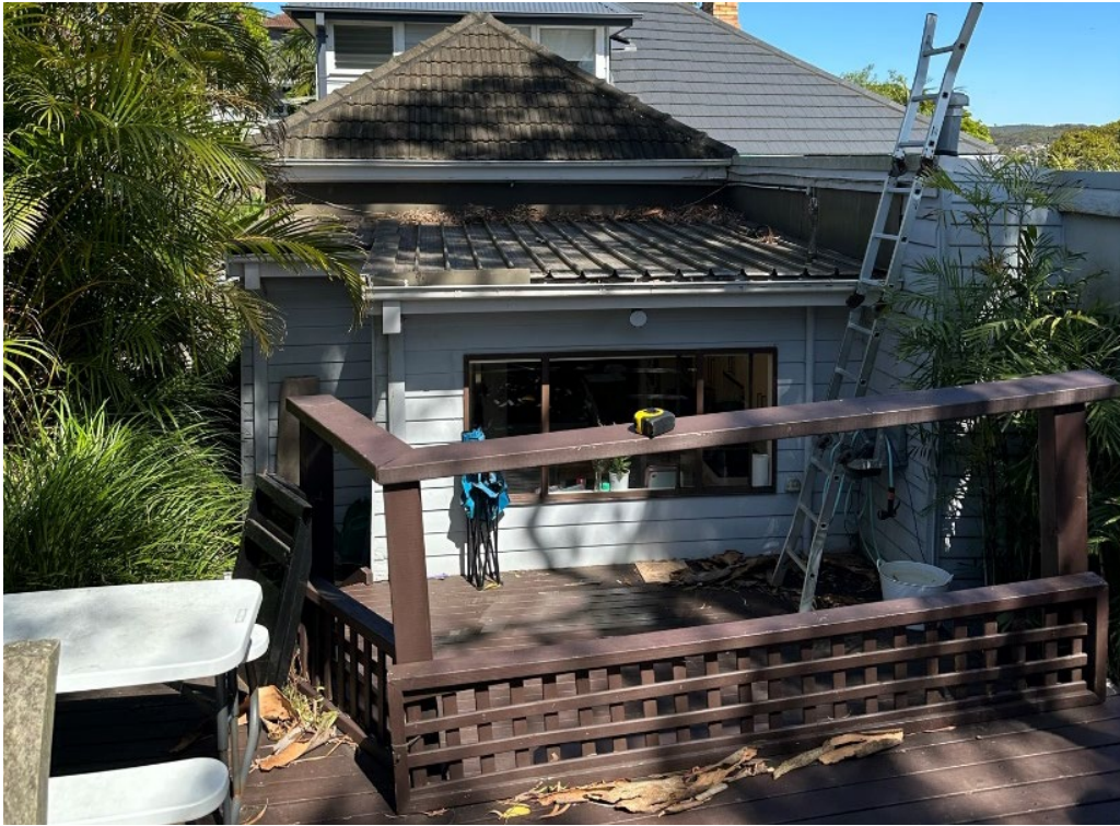
Figure 5. View of existing decks and rear of dwelling (existing kitchen/dining).
