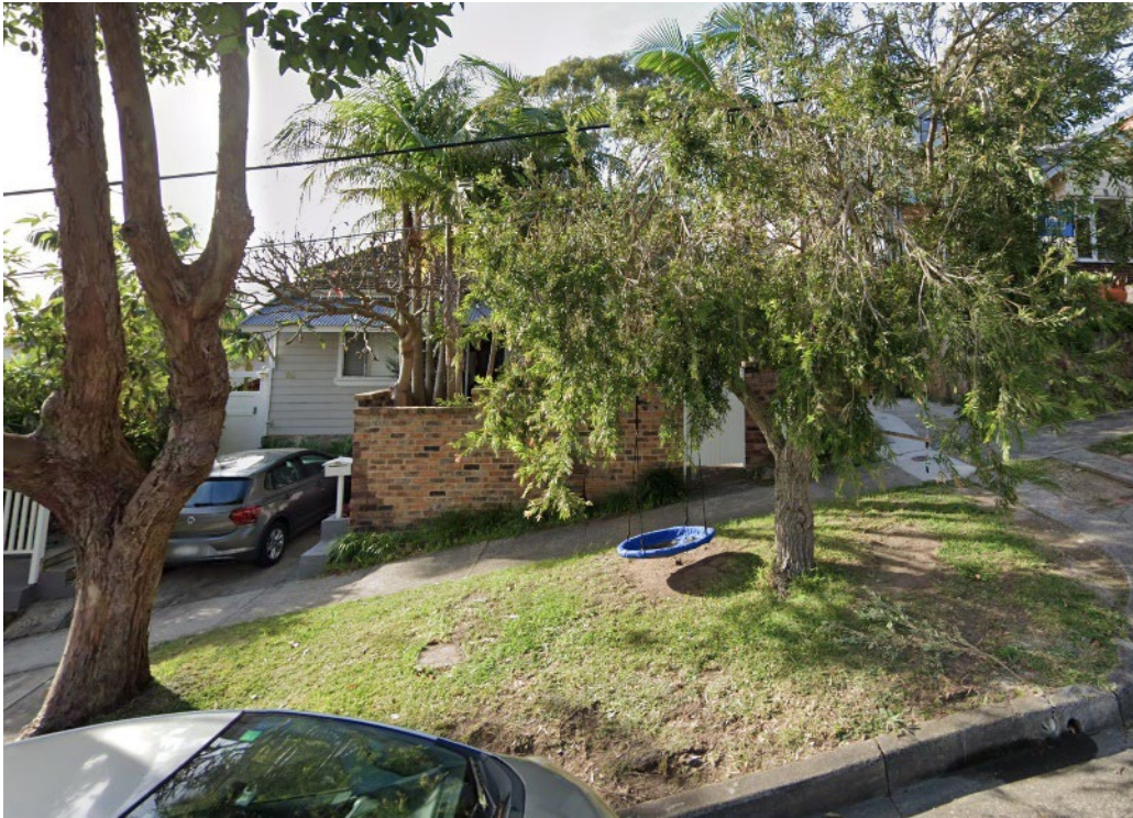
Figure 3. No.14 Bellevue Street (centre) – Street elevation (#16 left).
