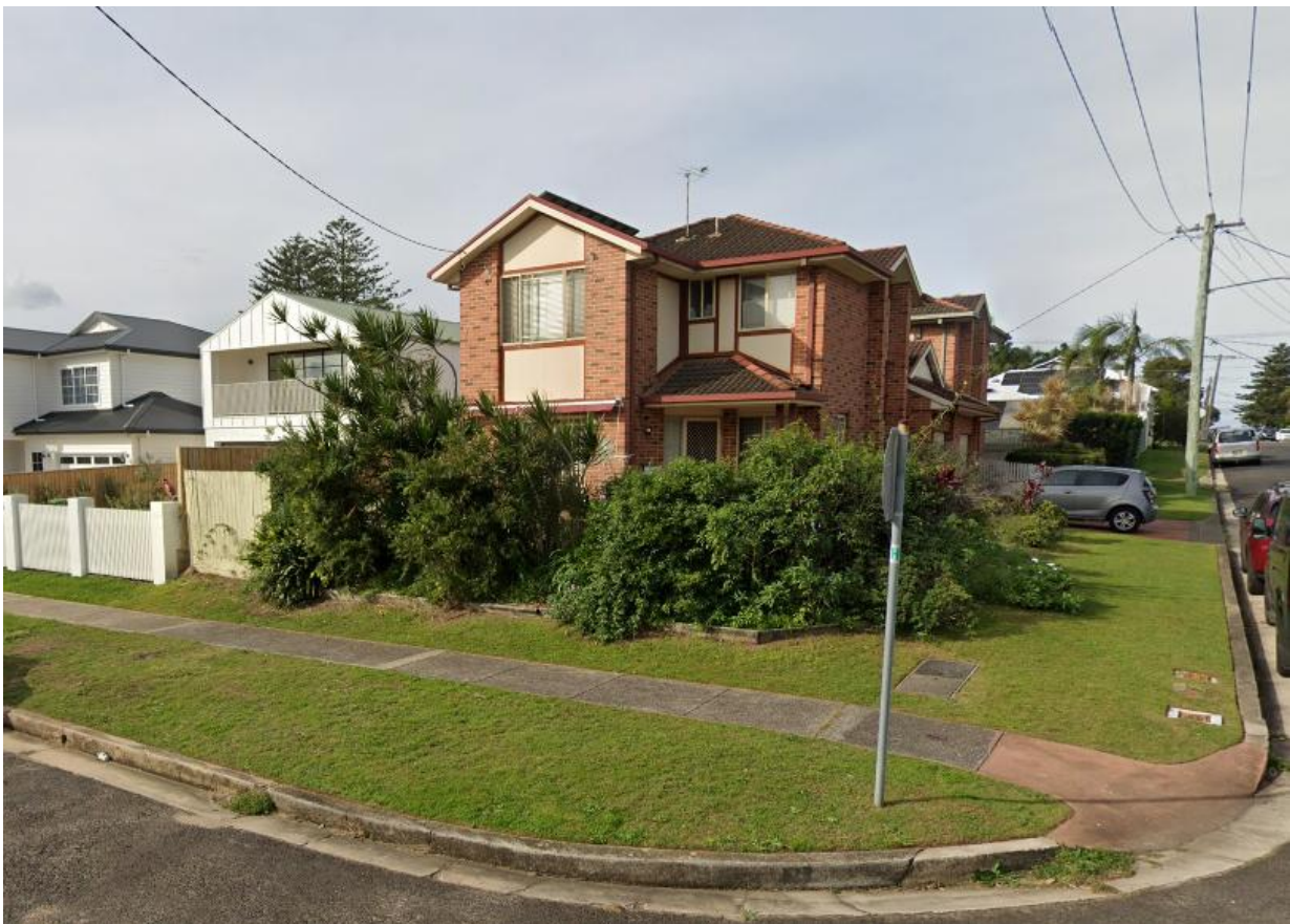
Image 3: Lisle Street frontage
