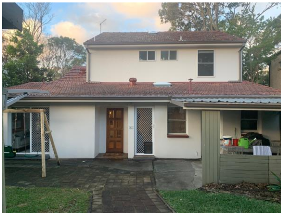
View looking north east; location proposed new window and door configuration to existing dwelling
