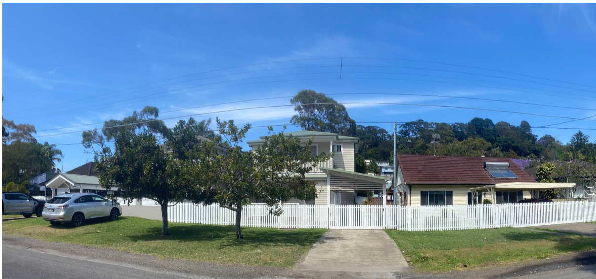
Image: Carports located at 21, 23 and 25 Narroy Road
