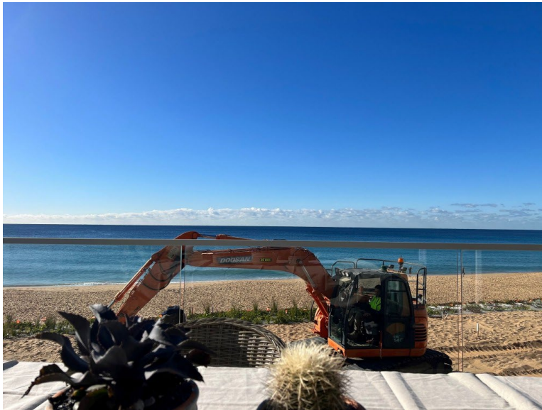
Figure 10. Sitting on the first floor deck, facing east over the rear boundary.
