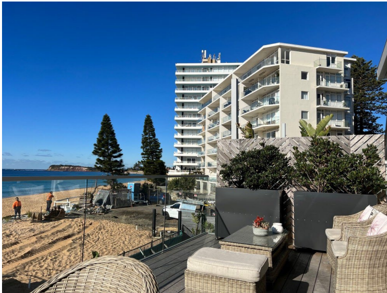
Figure 8. Standing on the first floor deck, facing south-east over the side boundary.
