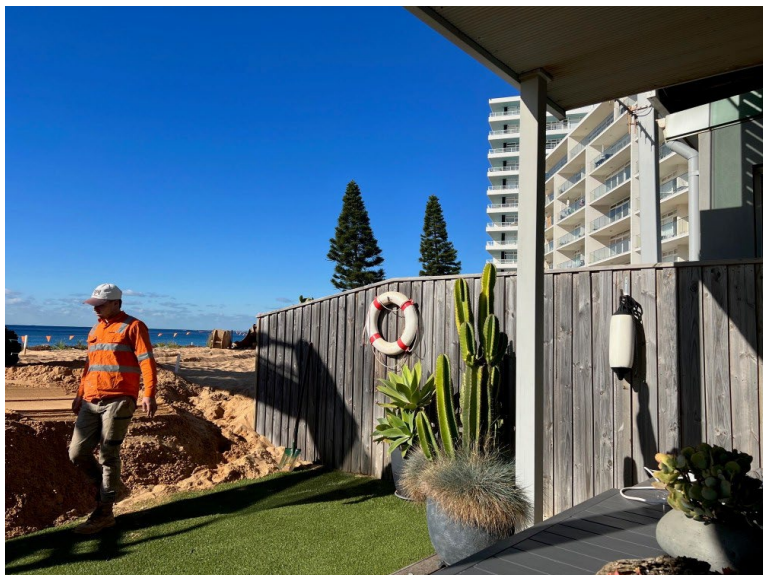
Figure 7. Sitting on the ground floor deck, facing south-east over the side boundary.
