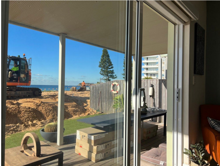
Figure 4. Standing in the ground floor living room, facing south-east across the side boundary.
