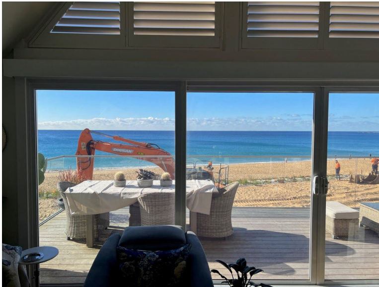
Figure 16. Standing in the living room on the first floor level, facing east over the rear boundary.
