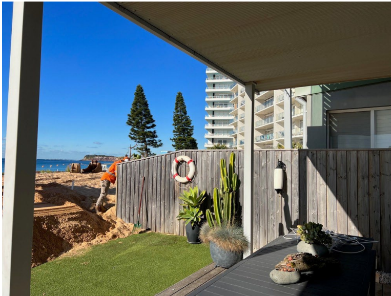
Figure 6. Standing on the ground floor deck, facing south-east across the side boundary.
