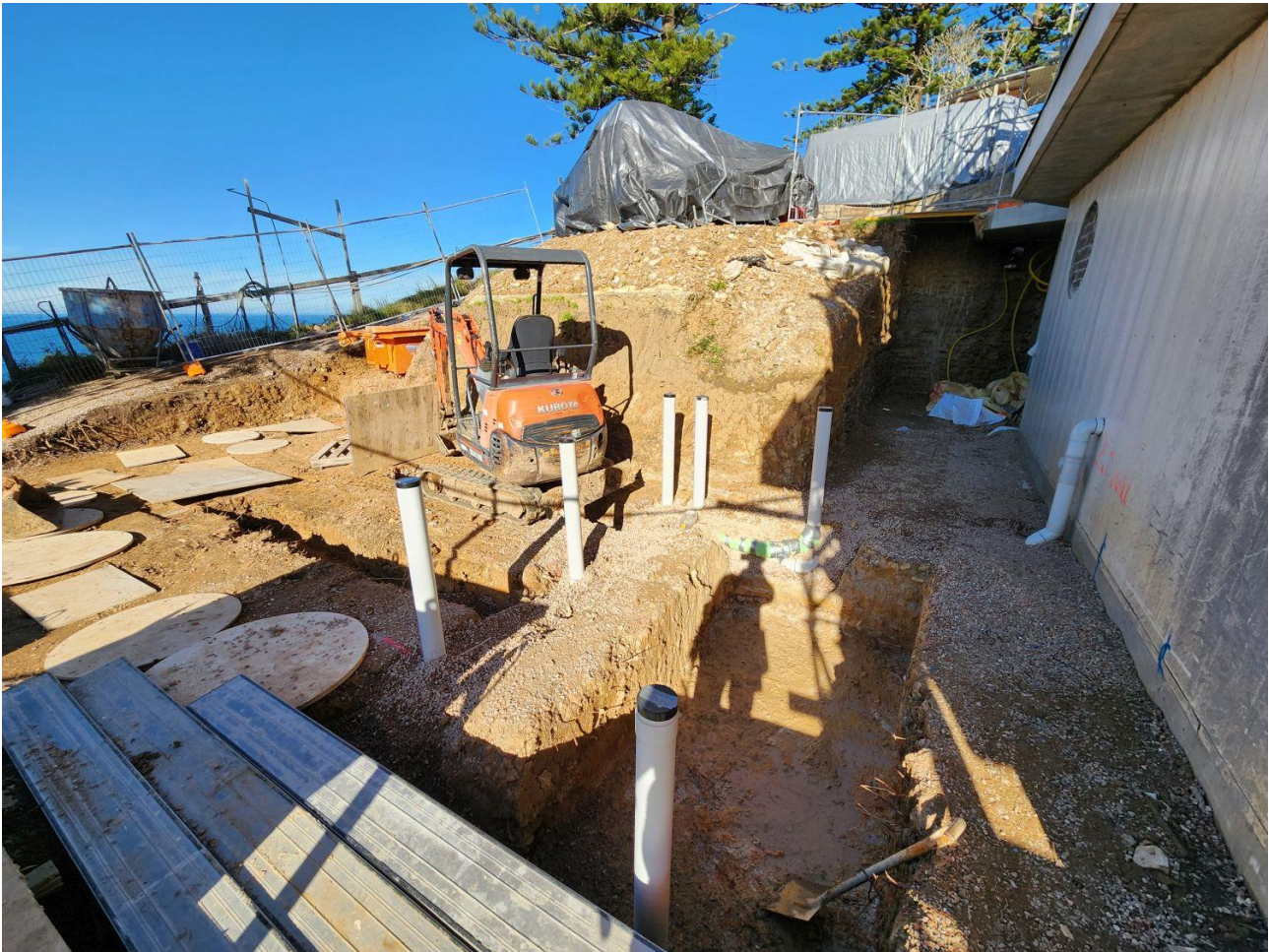
Photo of Inspected Area- looking south-east wards
