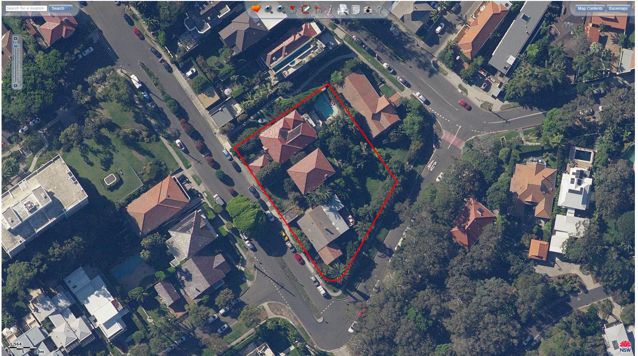
Figure 1-3: Close-up aerial image of project site.
