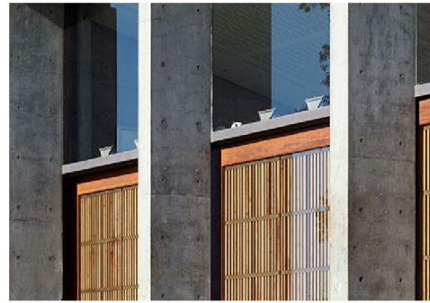
A – OFF-FORM CONCRETE GLENN MURCUTT, WENDY LEWIN AND REG LARK – ARTHUR & TYONNE BOYD CENTRE.
