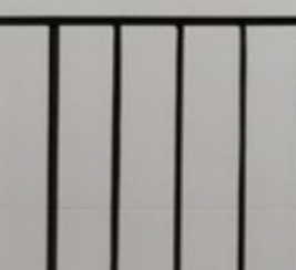
BAL01 BALUSTRADE STEEL BLACK POWDERCOATED
