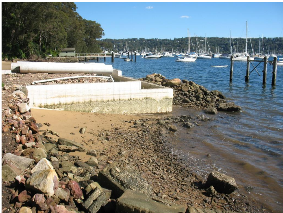
Figure 5. Foreshore: artificial sandstone retaining wall, foundation walls and pile of boulders (northern side). Four piles of the former jetty were present offshore.
