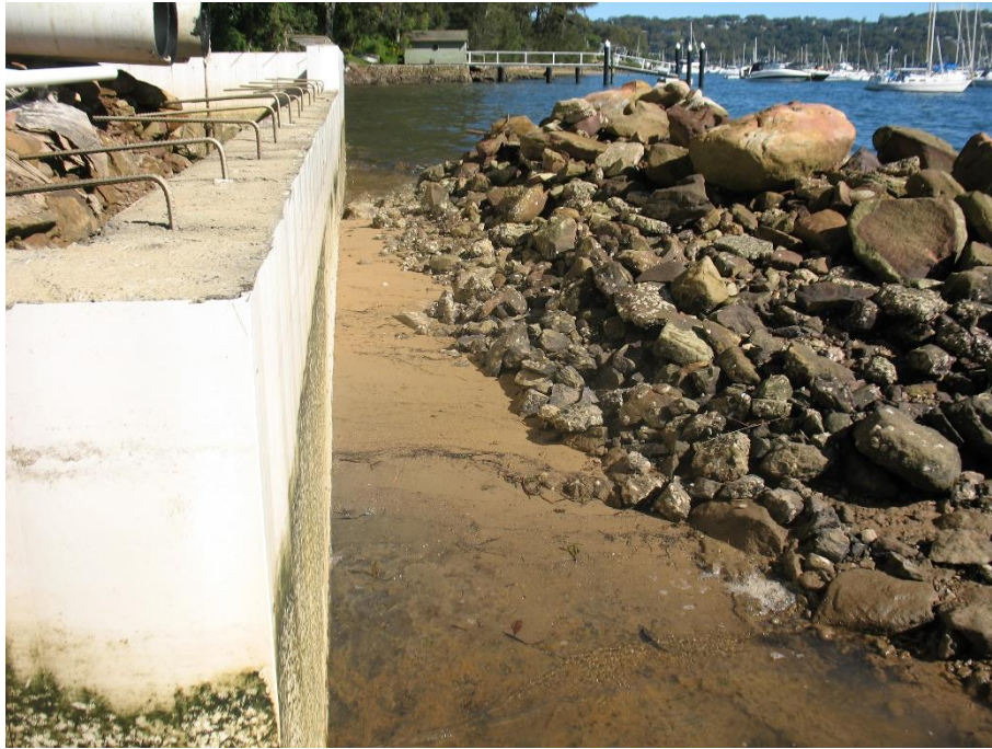
Figure 6. Foundation walls and pile of boulders (western side).
