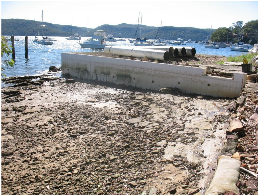
Figure 4. Foreshore: artificial sandstone retaining wall and foundation wall, natural sandstone platform (southern side).
