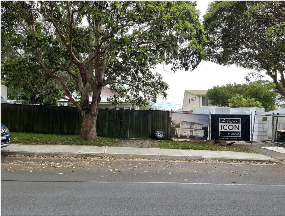
Figure 12. The subject site and dwelling under construction at 6 Freshwater Parade.
