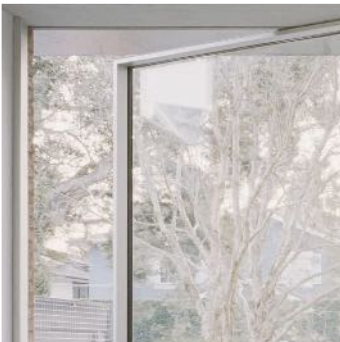
Window Frames - light colour aluminium
