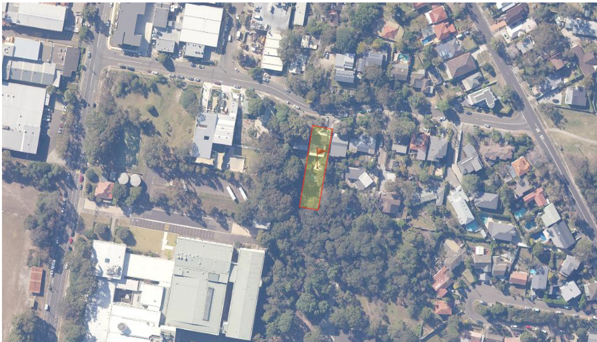
Image 2. Site location: 26 Orlando Road, Cromer NSW (© SIX Maps NSW Gov)
