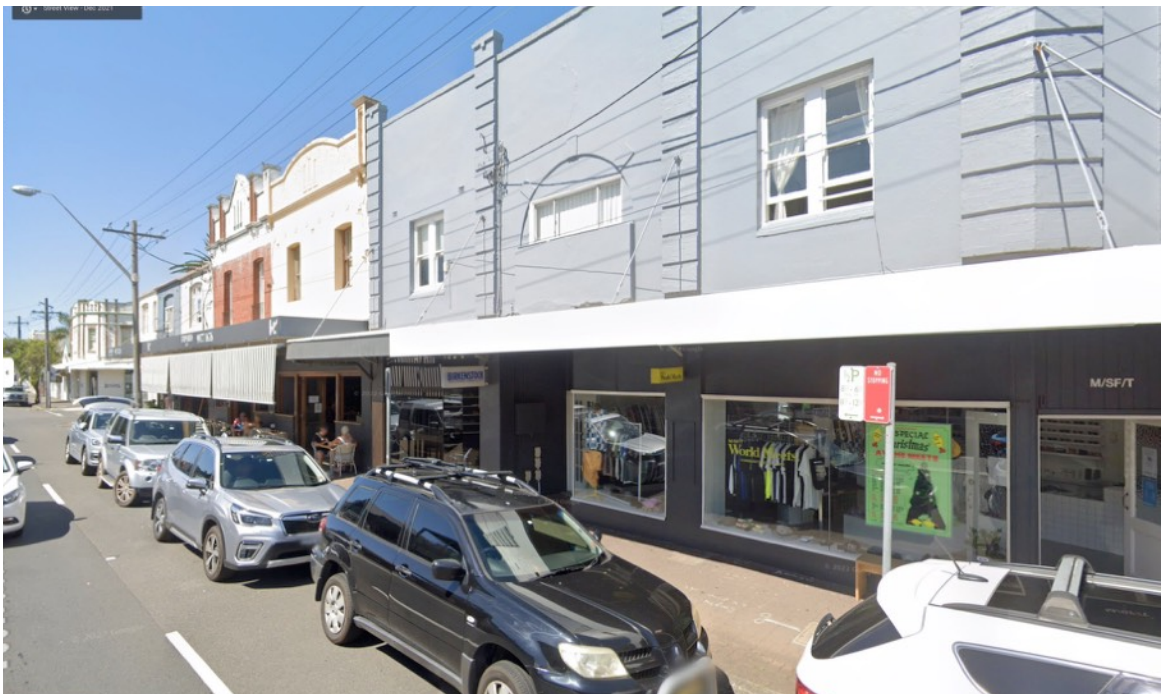
View of the commercial buildings in a contiguous row with original detail between Golf Parade and Rolfe Street.
