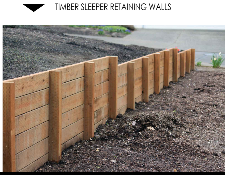
TIMBER SLEEPER RETAINING WALLS
