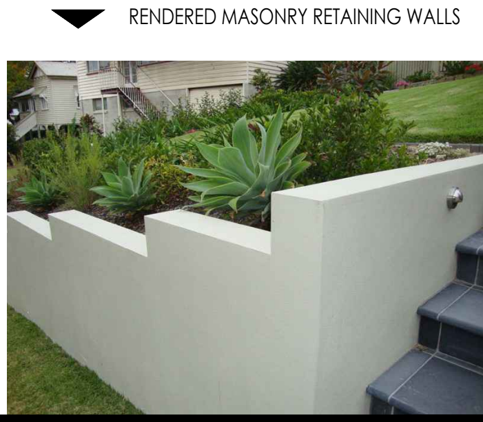
RENDERED MASONRY RETAINING WALLS
