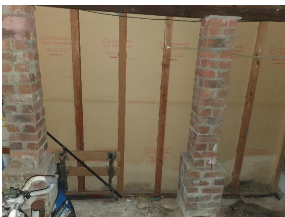
Photograph-1: Brick columns supporting western portion of the dwelling. View facing west towards the back of the timber rear laundry wall, that is proposed to be demolished.
