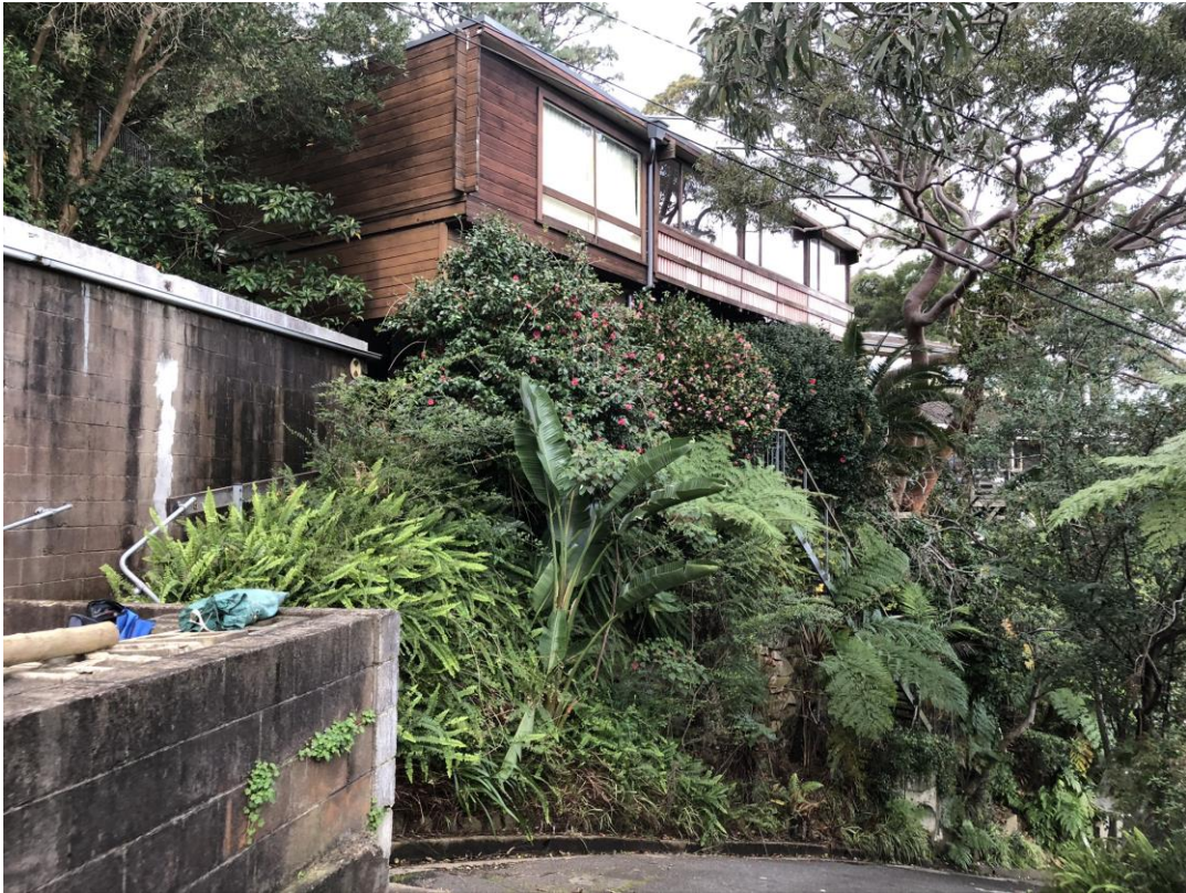
Figure 6. The dwelling viewed from the east
