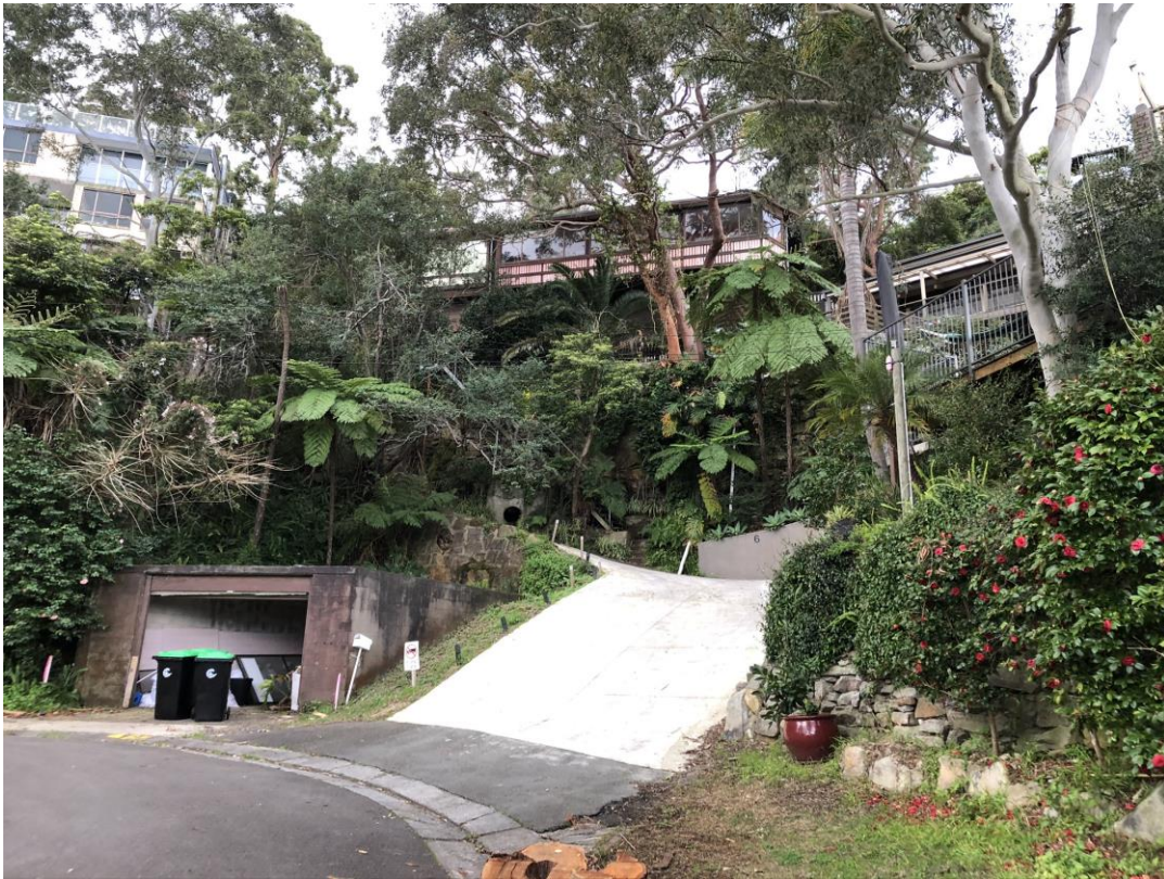
Figure 4. The dwelling viewed from Berrinda Place
