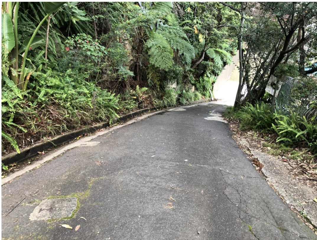
Figure 5. The existing driveway (ROW) providing access to the dwelling
