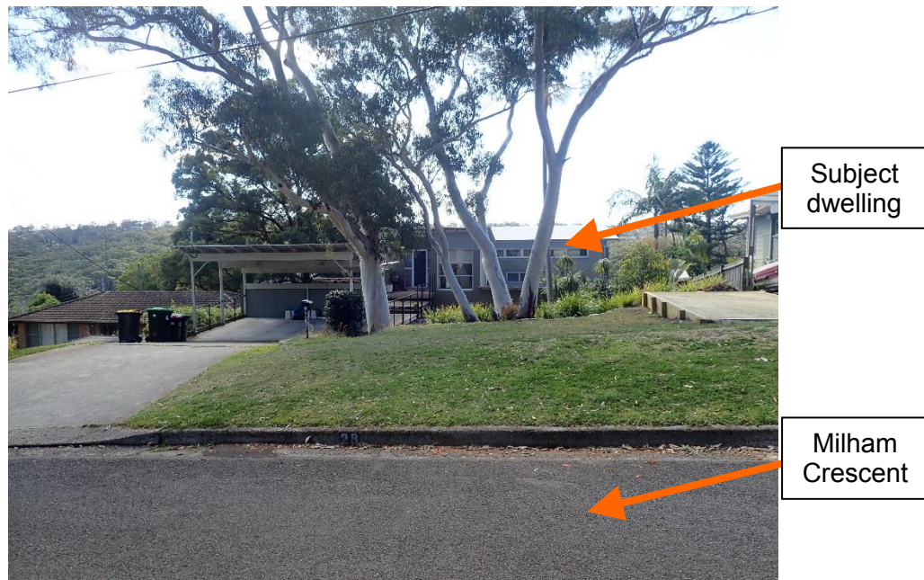
Photograph 01: View north from Milham Crescent toward the subject site
