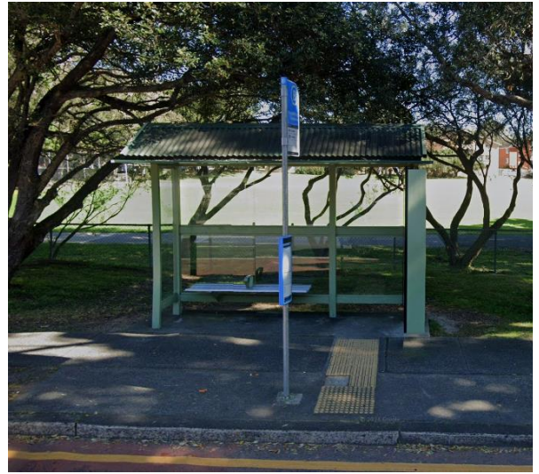
Figure 3 Existing J2 Bus Stop and Shelter on Pittwater Road, in front of 738 Pittwater Road, Dee Why
