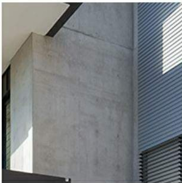
F_ OFF FORM CONCRETE
