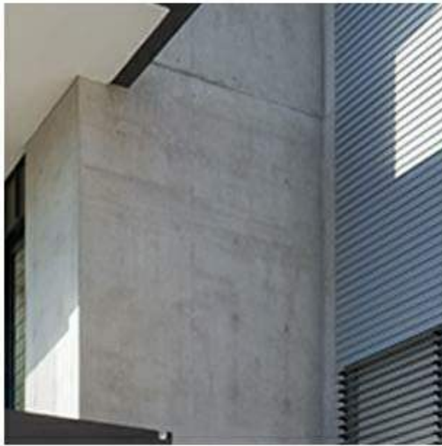
F_ OFF FORM CONCRETE
