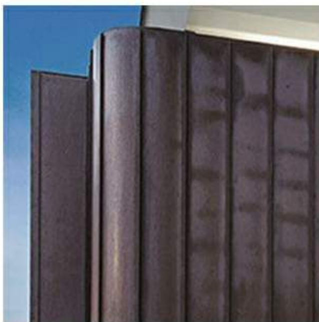
J_ COLOURED METAL CLADDING
