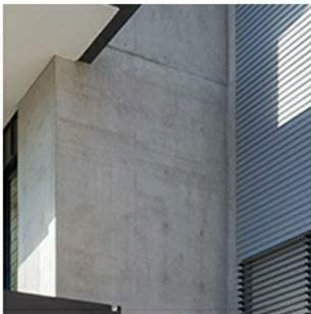
F_ OFF FORM CONCRETE
