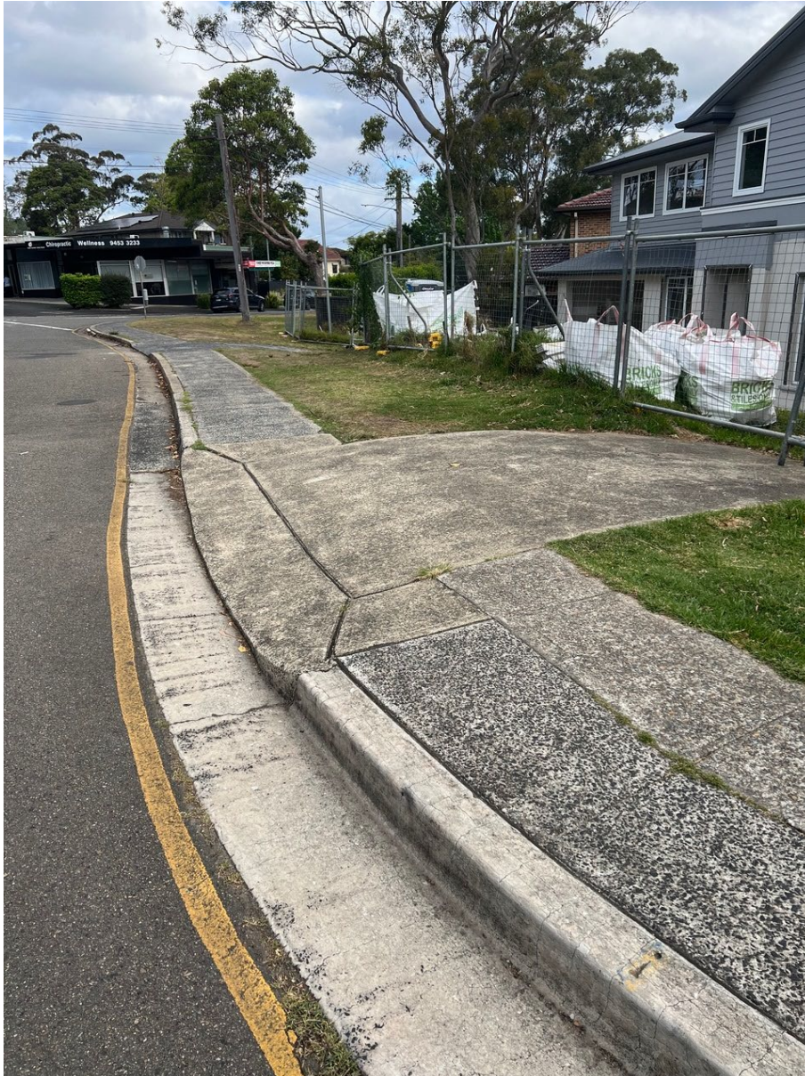
Figure 2 View South east along Arthur Street
