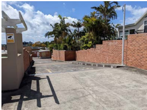
Figure 3 – Concrete paved driveway (suspended slab)
