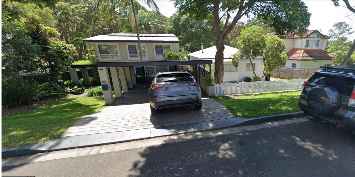
NO. 33 CONDOVER STREET- DOUBLE CARPORT TO THE FRONT.
