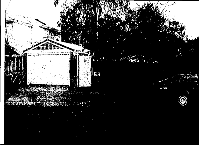
Street view of 10 Angle St with carport
