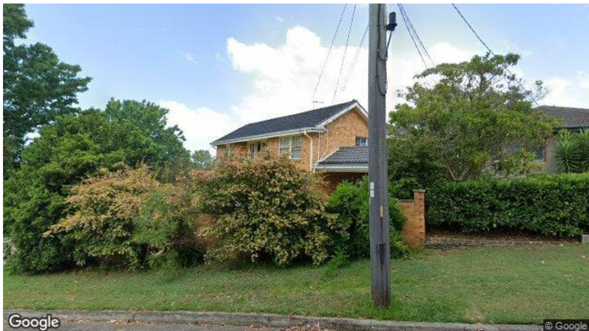
FIGURE 3: Street View, 1 DONEGAL ROAD, KILLARNEY HEIGHTS. Source Realestate.com. 3
