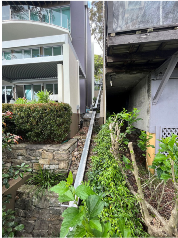
Photo 5: Below swimming pool viewing South & adjoining Inclinator rail.
