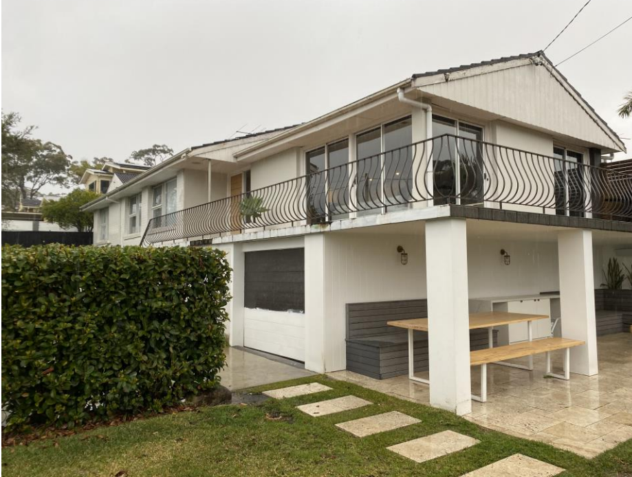
Figure 12. Looking south west, the existing balcony to be partially enclosed
