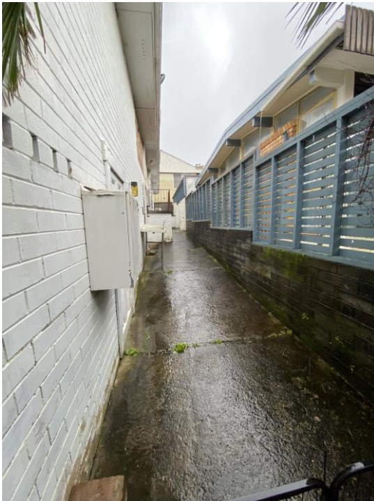
Figure 13. Looking south, the western side setback and adjoining dwelling at 3 Windermere Place
