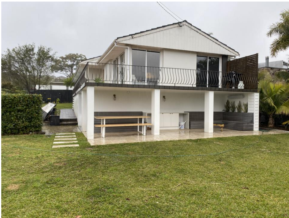
Figure 11. Looking south, the northern elevation of the existing dwelling (and the existing balcony to be partially enclosed)
