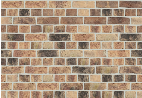
EXISTING BRICK WALLS
