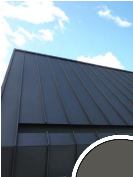
METAL ROOFING AND GUTTERS
