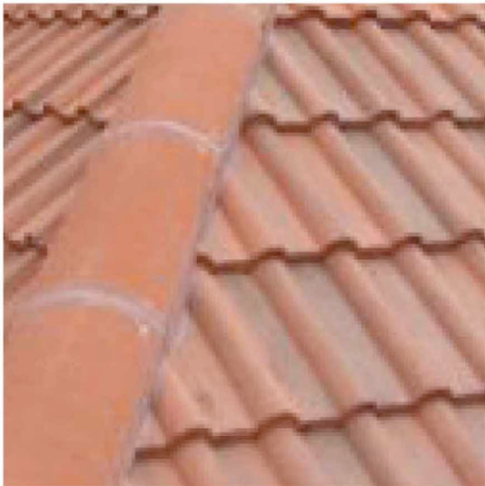
1. Existing roof tile.
