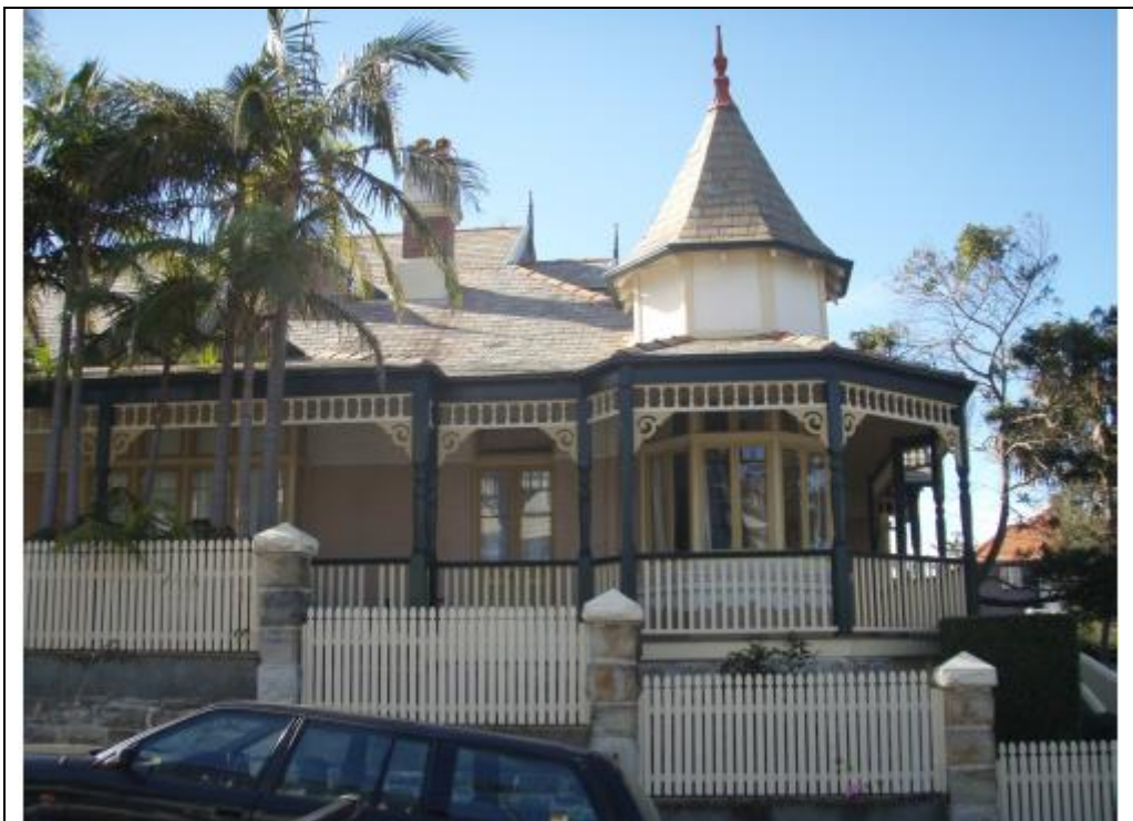
14 Camera Street – diagonally opposite the site. Heritage listed item
