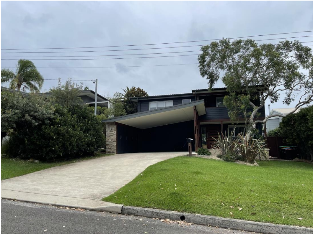
Figure 7 Existing carport on Elvina Avenue
