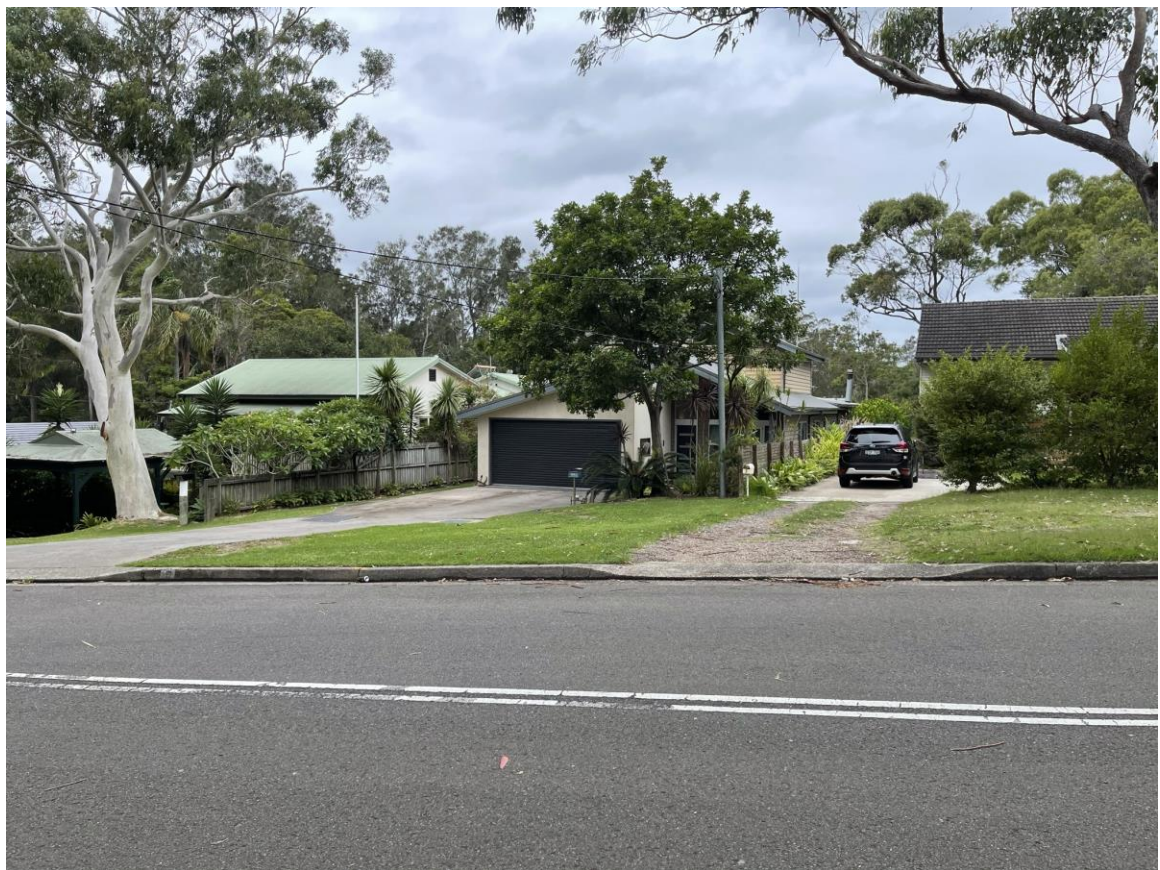
Figure 4 The site viewed from Elvina Avenue
