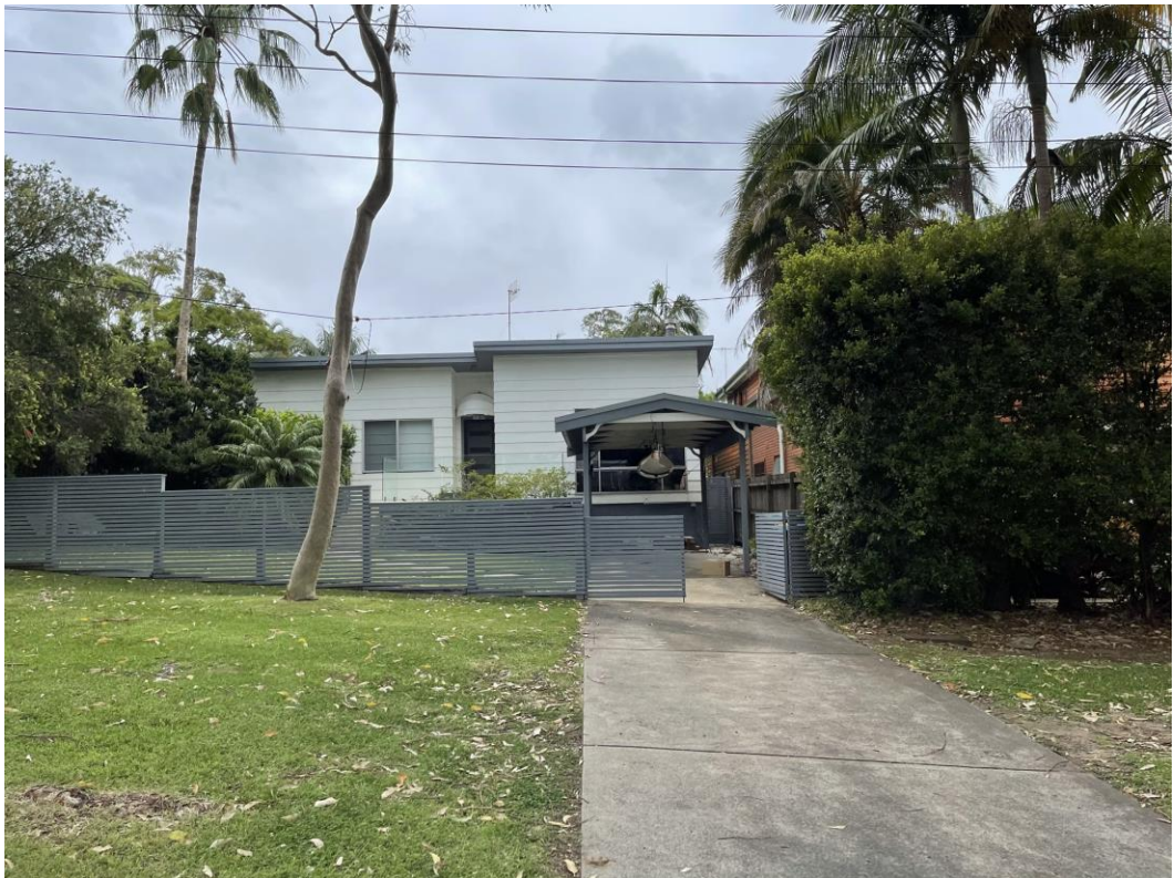
Figure 8 Existing carport on Elvina Avenue
