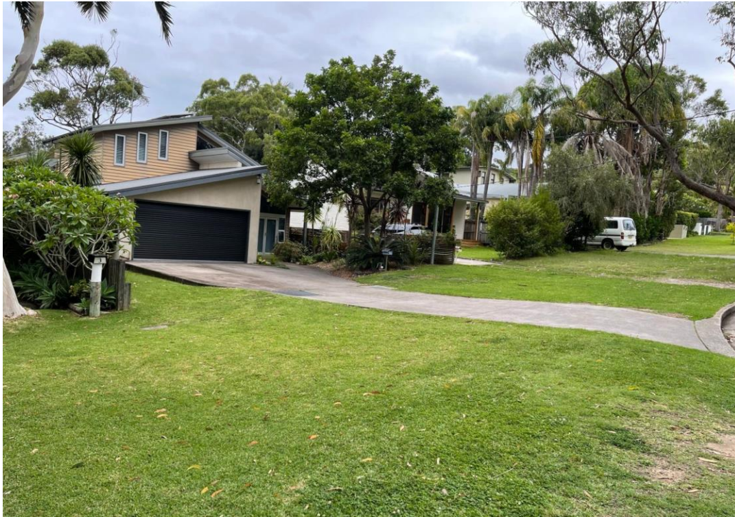
Figure 5 The existing driveway including the council verge
