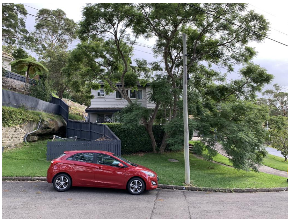
Fig 5: View of existing dwelling, looking south-west from Ashdown Place cul-de-sac
