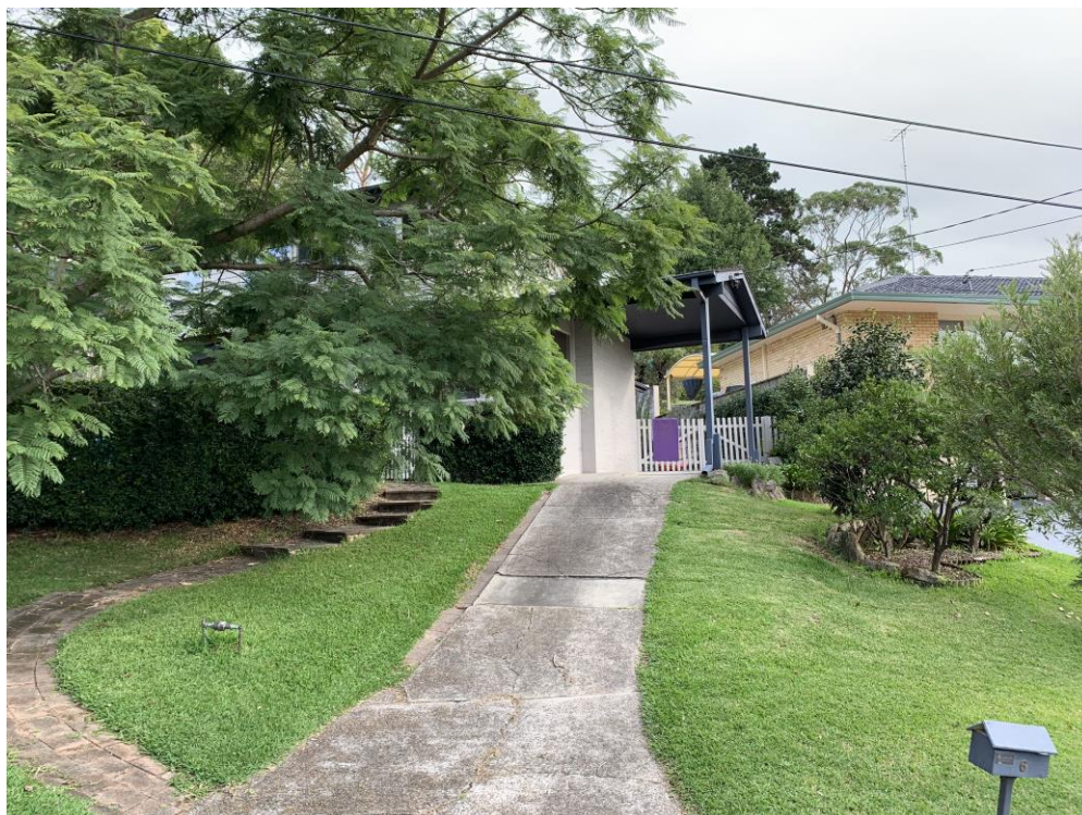
Fig 2: View of existing dwelling and existing carport (to be enclosed), looking south from Ashdown Place
