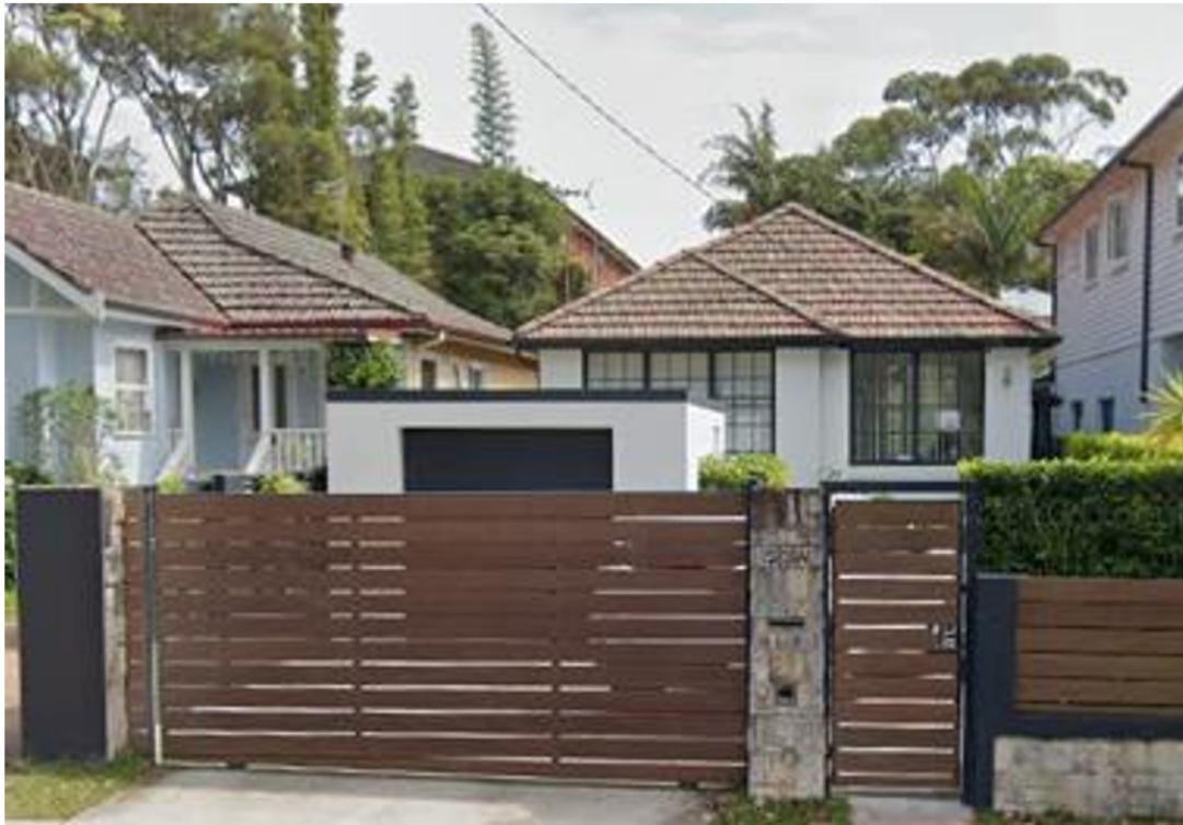
Existing Dwelling House - View from Wyuna Avenue
