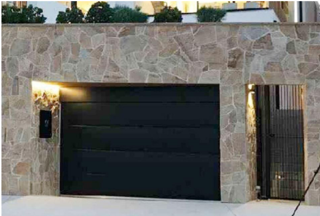
Sandstone to garage wall
