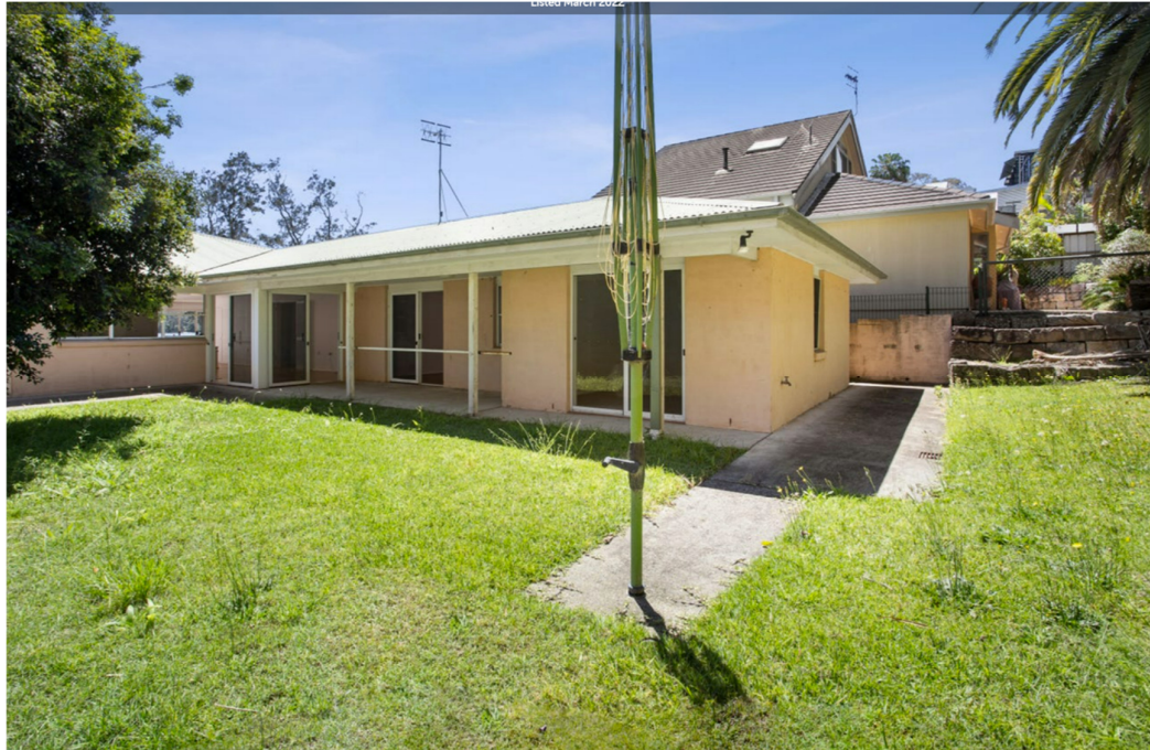
Figure 3 – showing the existing site as viewed from the rear
