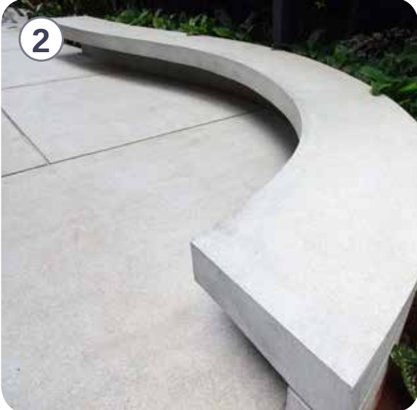
Concrete seating wall
