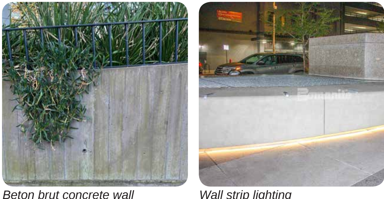
Beton brut concrete wall Wall strip lighting
