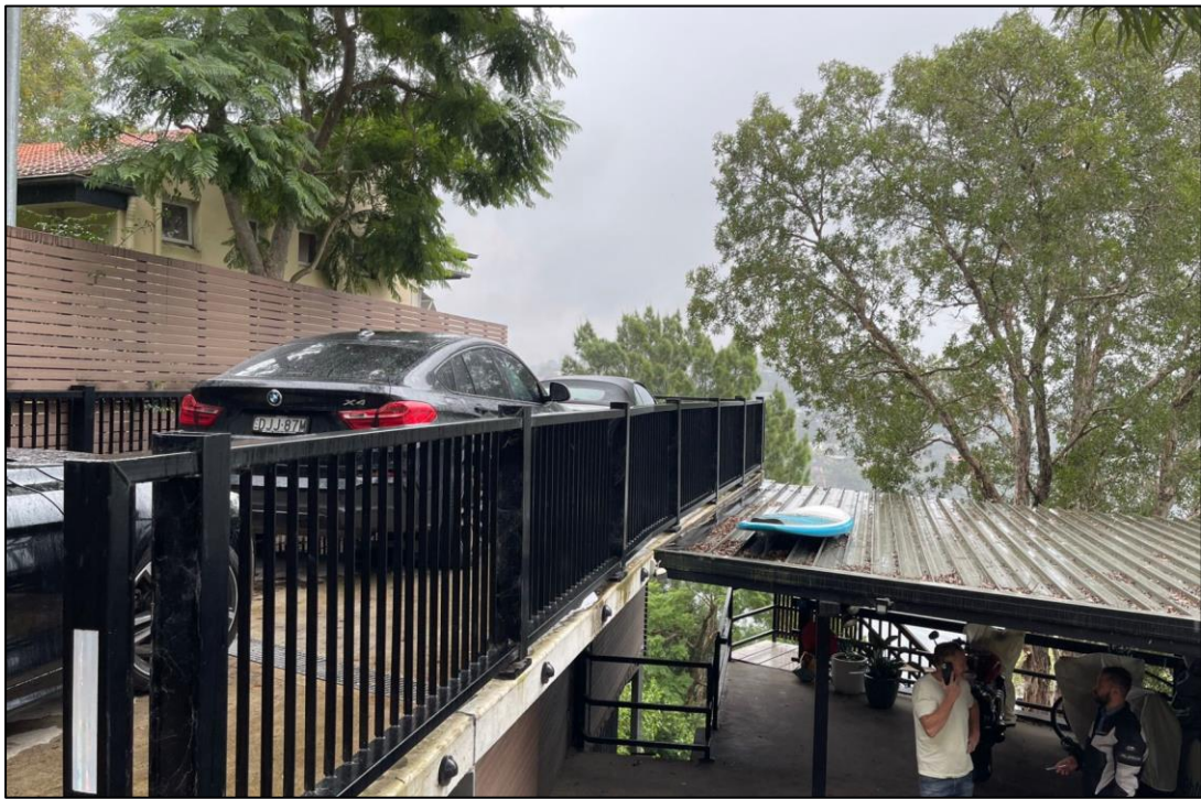
Figure 6. The adjoining property and suspended driveway to the south.
