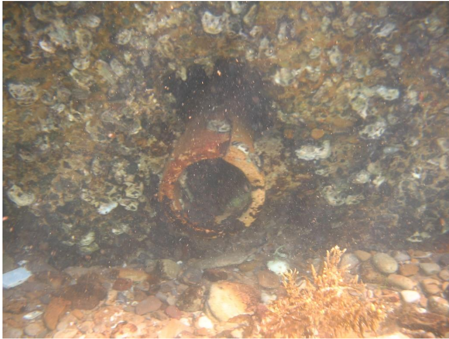
Figure 4. Foreshore: artificial concrete seawall and a drainage outlet (to be upgraded). Structures were colonised by oysters, various gastropods and turfing algae.
