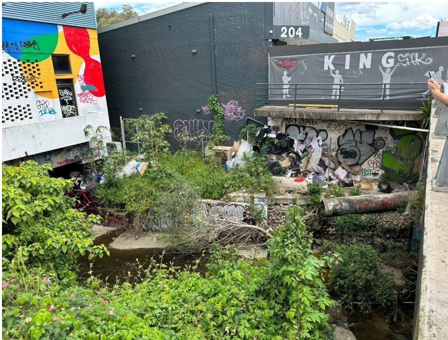
Photo 3: Open concrete channel with sparse vegetation before closed channel under adjacent building
