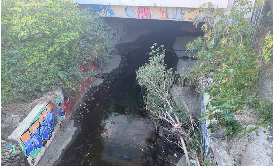
Photo 1: Concrete Lined channel adjacent to site
