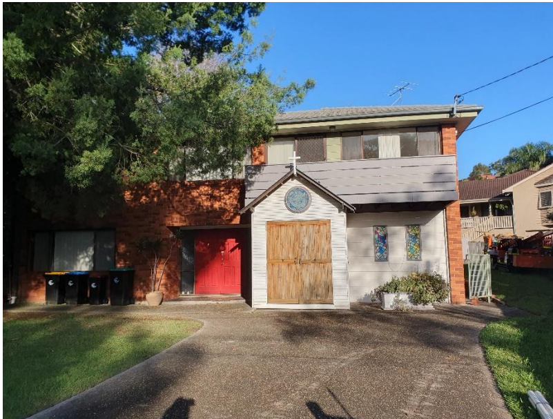
Photograph-2: Front of existing dwelling at No.1803a Pittwater Road. View looking west.
