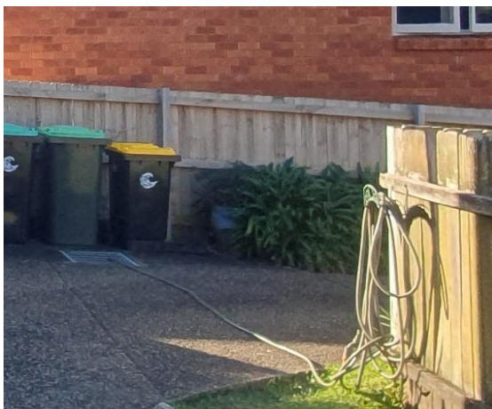
Photograph-7: Water tap leakage. View looking north front the front of the rear block.
