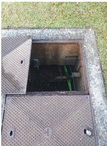
Photograph-5: Service at the road reserve. View looking down west.
