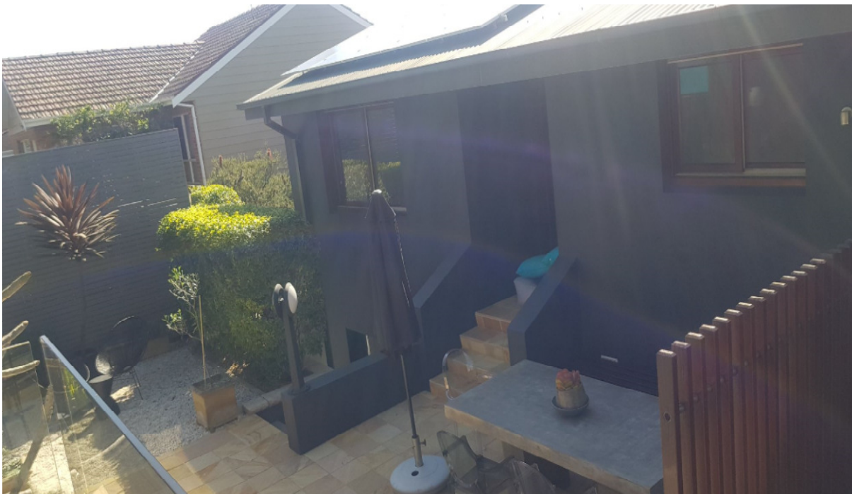
Photo showing the back of the subject dwelling and the privacy screen to No 12 Lancaster Street.
