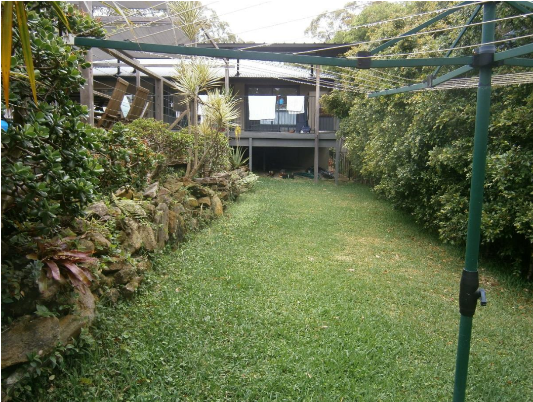
Views of the existing south west side of the house/location of the proposed addition.
