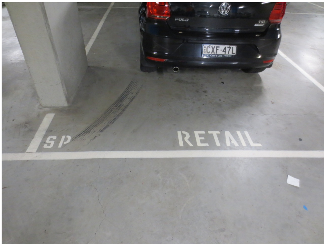
Figure 4 – Staff Parking Space Line Marking
