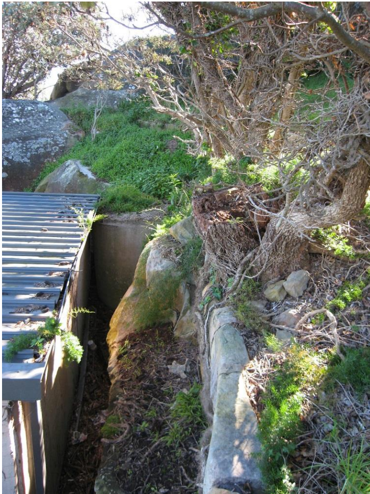
Figure 5: Trees 4 and 5, located at top of old sandstone wall. Tree 4 are stems growing out of decayed stump.
