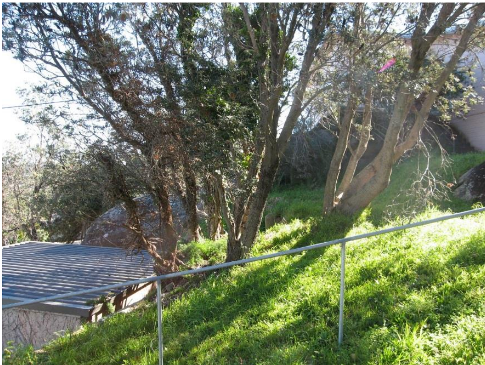
Figure 4: Group of trees Trees 2, 3, 4 and 5. Note Tree 2 uphill, leaning, failed root plate to south side.
