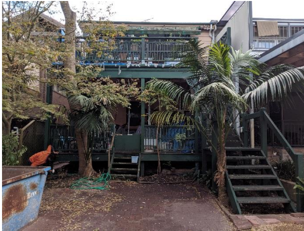
Figure 2. Photo of the rear of the property with the existing two-storey deck.
