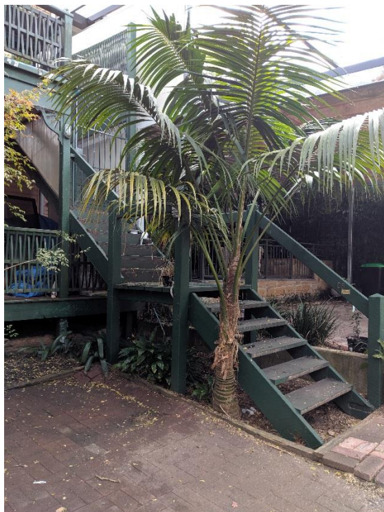
Figure 10. Existing stairs to the upper level of the deck and area where the eastern footing will be installed.
