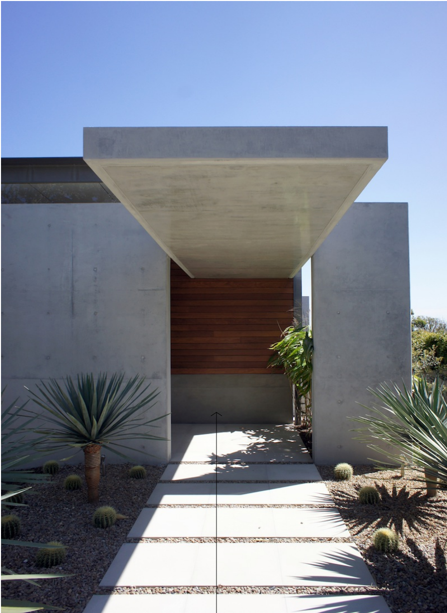
RN: Concrete render finish (external walls)
