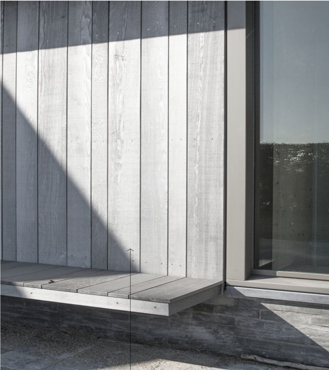
TC: Hardwood timber cladding (external walls)
