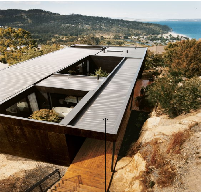
RS: Roof sheeting
