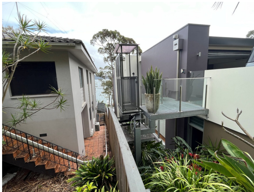
Photo 2: Elevated adjoining carriage and landing station & intended path of proposed Inclinator.
