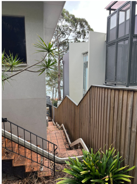
Photo 3: Fence on common boundary.
