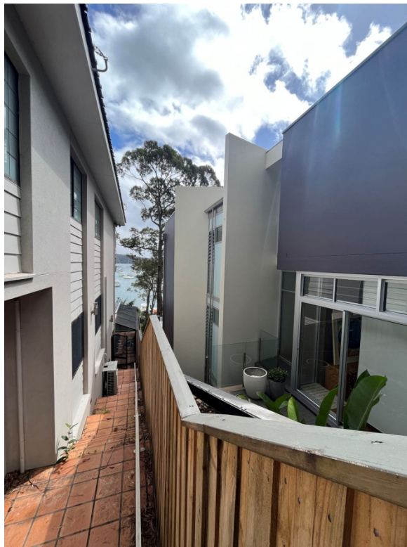
Photo 4: Inclinator path and adjoining residence.
