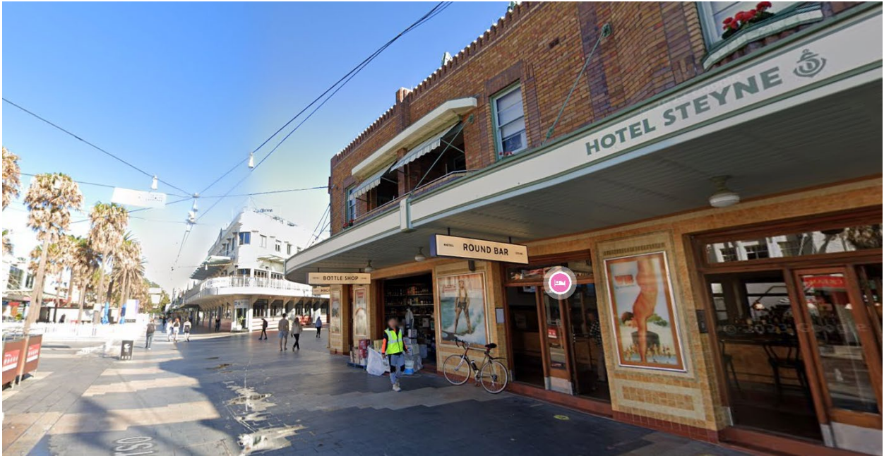
FIGURE 4: PHOTO OF HOTEL STEYNE AND NEW BRIGHTON HOTEL OPPOSITE THE SITE
