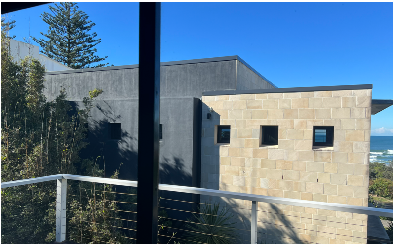
Figure 9. Standing in the kitchen, facing north-east, at 16 Bassett Street
